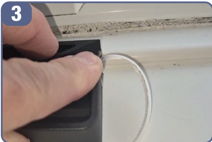
Push the SafestCut along the sealant that is to be removed
