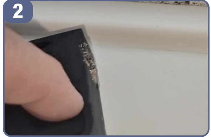
Press the bladed corner of the SafestCut into the sealant at a shallow angle until the unit is against both surfaces
