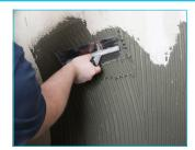
Spread the adhesive according to the manufacturers instructions. Use a Vitrex Notched Adhesive Trowel for the best results. Spread about 2 square metres at a time.
