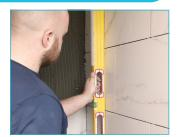
Check with a spirit level that the tiles are square. If using Vitrex LASHXL, use Lash Pliers to tighten the Wedge into the Spacer. Once dry, Wedges can be removed.
