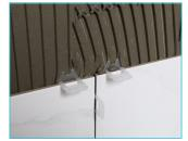
Start laying your tiles, adding Vitrex LASHXL Spacers and Wedges or use a choice of Vitrex Tile Spacers.
