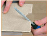
To smooth sharp and uneven edges, use a Vitrex Tile File. File away from the glazed edge.
