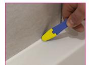
When the tiled surface joins another surface, apply silicone sealant. Use a Vitrex Flexi-Tip Sealant Smoother for a perfect watertight seal.
