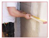
Ensure the surface is as flat as possible. Use a spirit level to ensure the wall is level.
