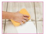
Use the Vitrex Dual Purpose Grouting Sponge to remove excess grout. When dry, polish with a soft cloth. The Vitrex Grout Sponge is also perfect for keeping your tiles clean during installation as well as after.
