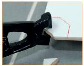
Use a Vitrex Tile Nipper to make awkward small cuts or nibbles until the desired shape is achieved.
