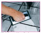
Work the grout in well using a Vitrex Grout Float or Spreader. Again, cover about a square metre at a time.
