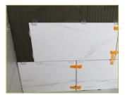
After the tiles have been laid using Vitrex Lash Levelling System, you will need to cut the remaining tiles to size.
