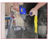
Mix the adhesive prior to placing the tiles on the wall. You can use a Vitrex Power Mixer. Follow adhesive instructions.
