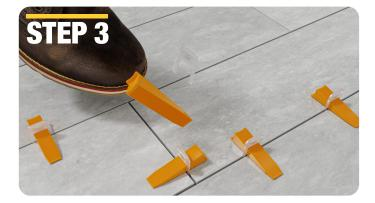
Let the adhesive dry as required by manufacturer's instructions. Simply kick the side of clips in the direction of the grout joints to snap them off or use a non-marking, rubber mallet. Keep reusable wedges for your next project.
